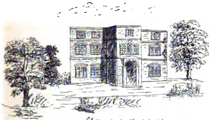
Clifton Hall (South Front)
